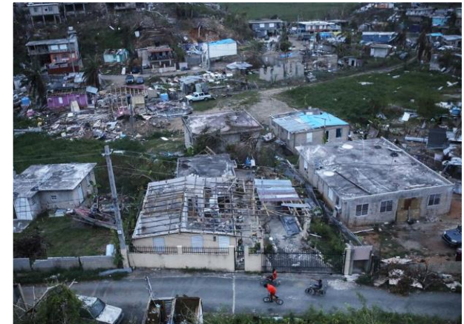
Figure 2: Storm damage from Hurricane Maria in Puerto Rico. Credit: Mario Tama, Getty Images.
